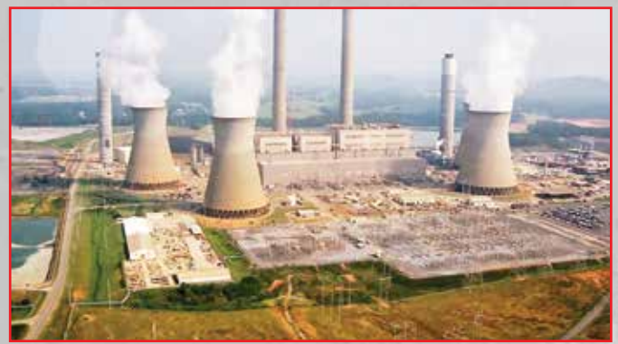
Matarbari Power Plant
